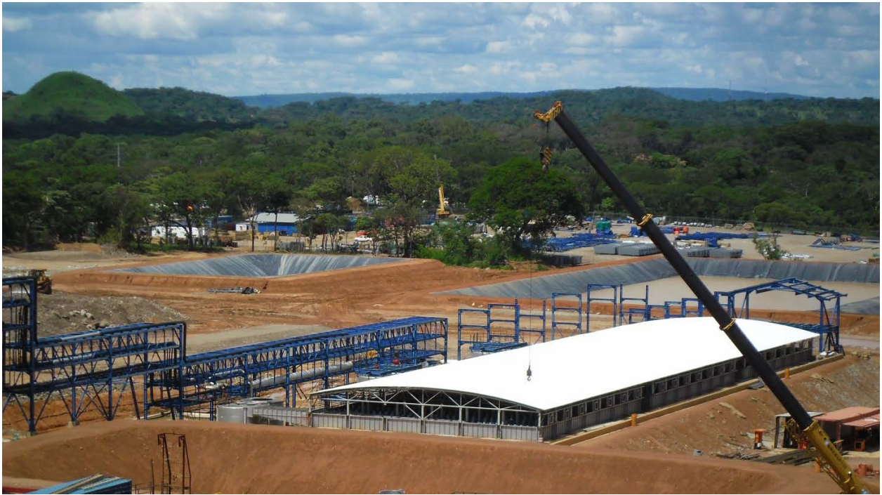
Solvent-extraction area 95% complete, with ponds containing first leached solution
