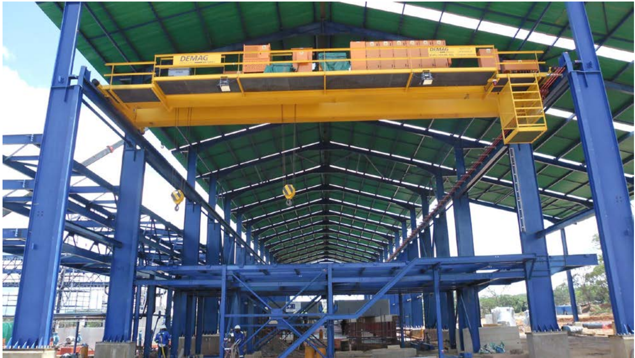
Electro-winning tankhouse 87% complete
