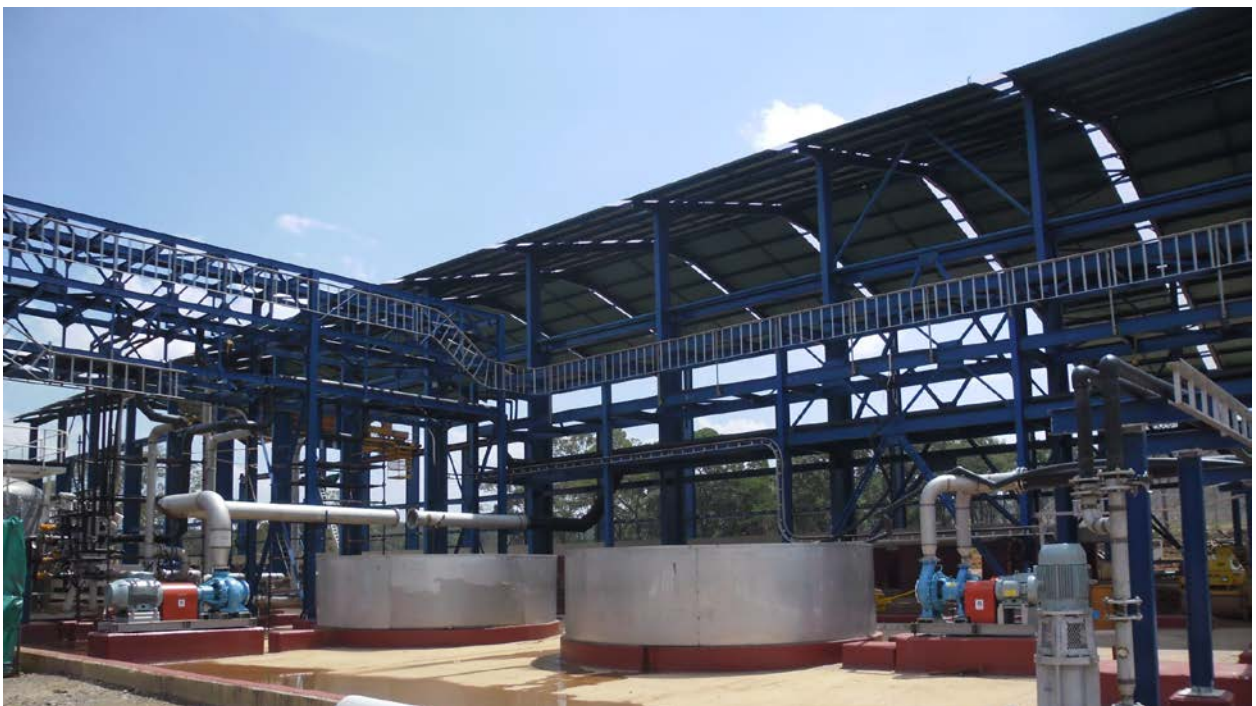
Electro-winning tankhouse 87% complete
